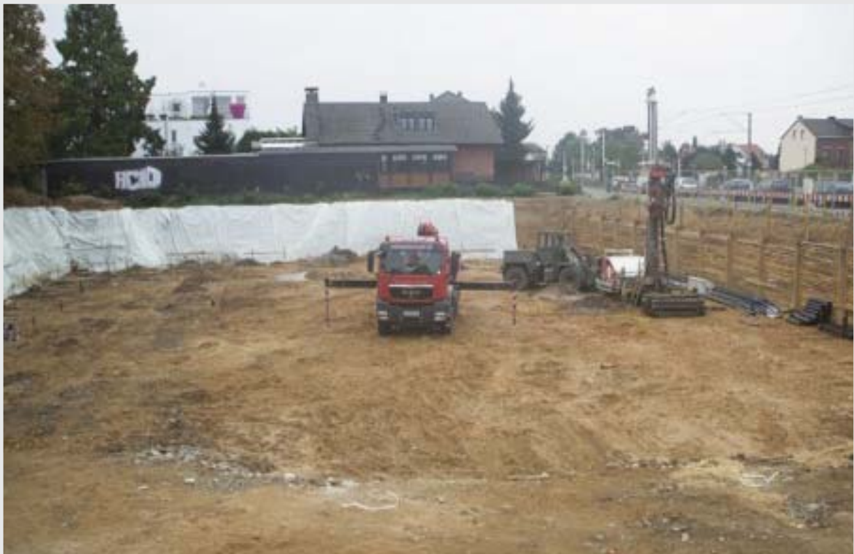
Installation of the GEOKOAX probe underneath the building.
