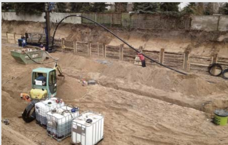
Figure 3: Installation of GEOKOAX probes below the building complex. (Foto: GEOKOAX GmbH)
