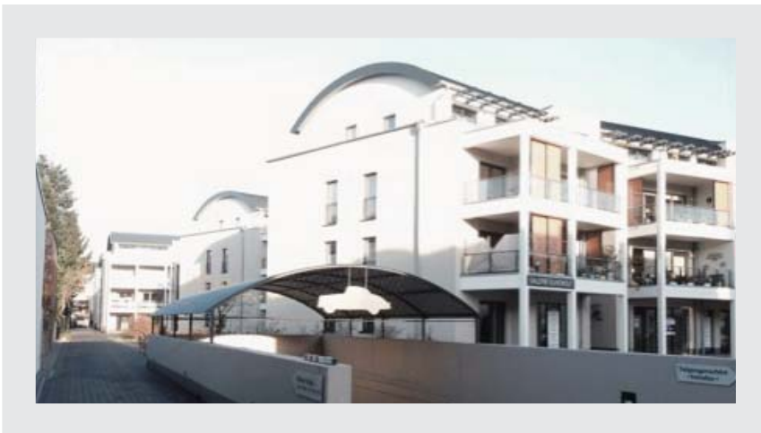
Figure 4: The completed residential and commercial buildings with rounded tent roofs. (Foto: EnergieagenturNRW)
